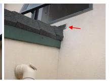
No Mechanical Head Flashing Above Vent Grille
